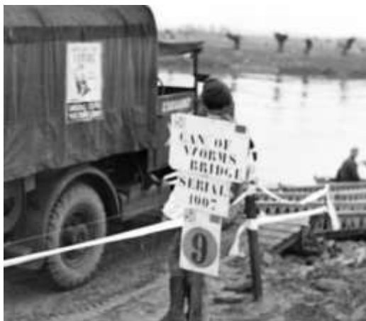
'Can of Worms Bridge'
